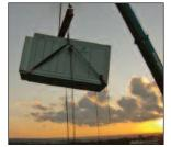
installed a CHP engine to cover the continuous demand for electricity and hot water. The 238 kWe plant uses natural gas to fire the CHP engine, recovering the waste heat emitted during the electrical generation process. The retrieved thermal energy is in turn
