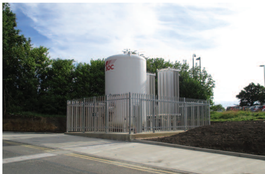
'Turnkey' installation of a medical gas supply system and pipeline by BOC – 'before' and 'after'.
